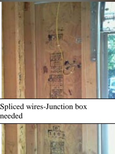
Secure wires in garage
