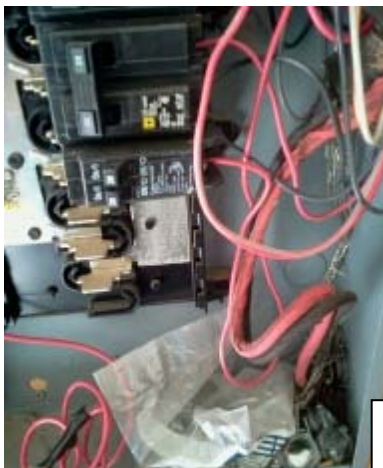
Recommend not storing parts in main panel
