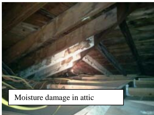
Moisture damage from Main Bath
